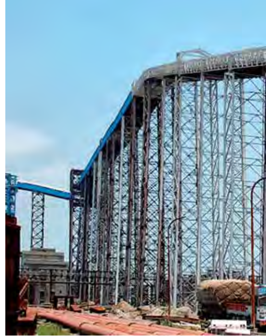
Extra Hi-Level Coal Conveyor for 3 x 500 MW Vallur TPP, Tamil Nadu
