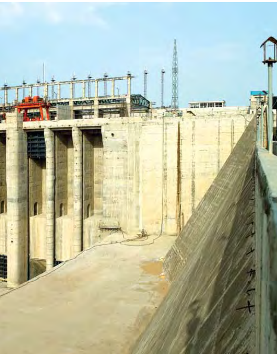
Intake Channel for 3 x 105 MW TONS HEP Tailrace, MP
